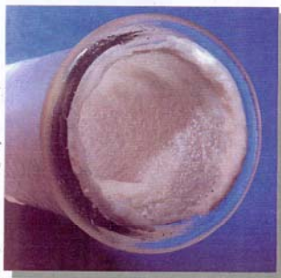
Hydrate deposition on a pipe wall.
